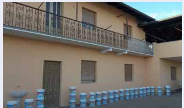
External facade of a house at Stroppiana (VC)
