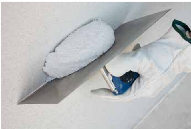
Application using a smooth-edged trowel
