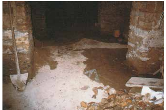
Photo n°1 - Cellar in Senigallia (AN) - Prior to renovation
